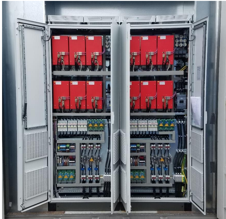
Figure 1: Example of two cabinets installed in a container
